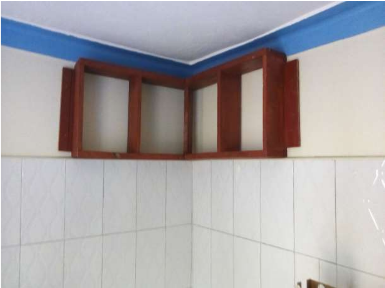
Renovated internal wall with Ceramic tiles and a file shelf
